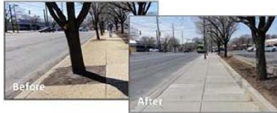
Sidewalk Improvement Projects: Flower Ave. to Greenwood Ave. (2010) Greenwood Ave. to Arliss St. (2011)
