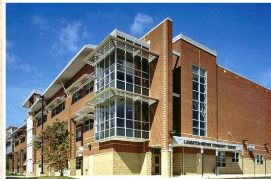
Langston-Brown School/ Community Ctr (LEED Silver)
