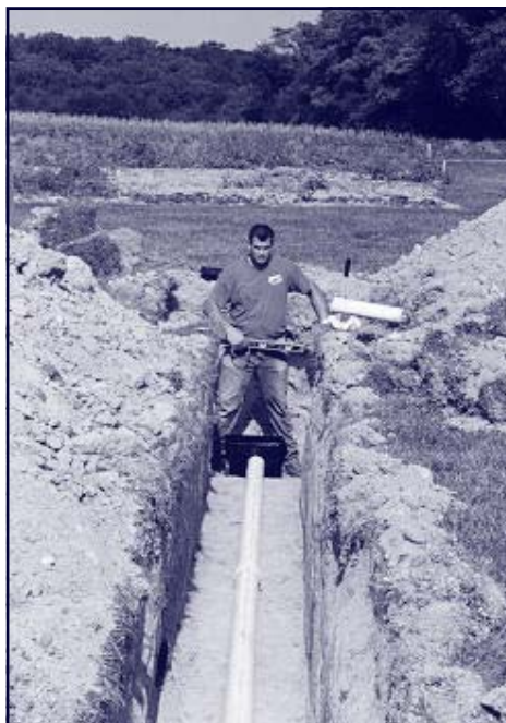
A worker prepares a trench and distribution box.
