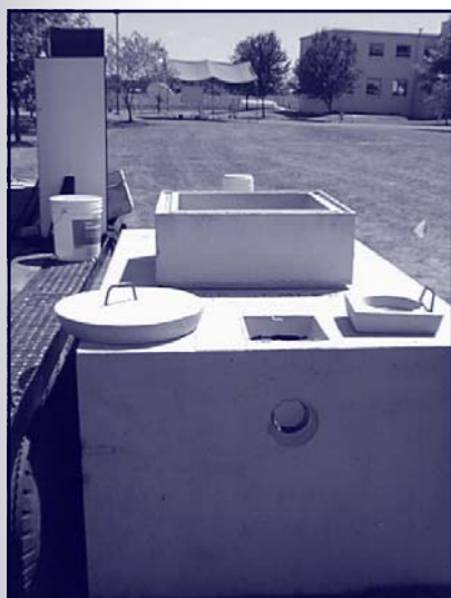
A two compartment tank is prepared to be set into the ground.
