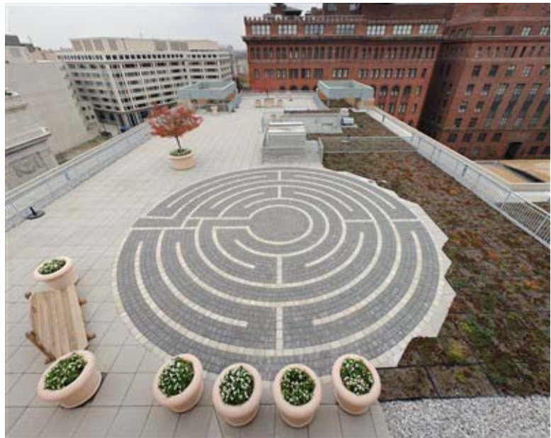
WRI green roof (Source: www.apabuilding.com )
