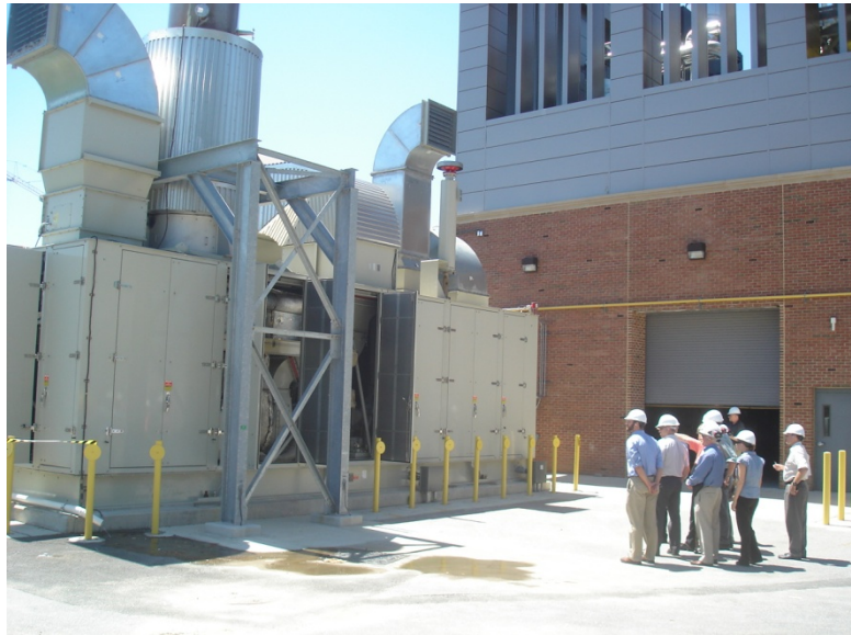
COG tour of White Oak combined heat/power and district energy facility.
