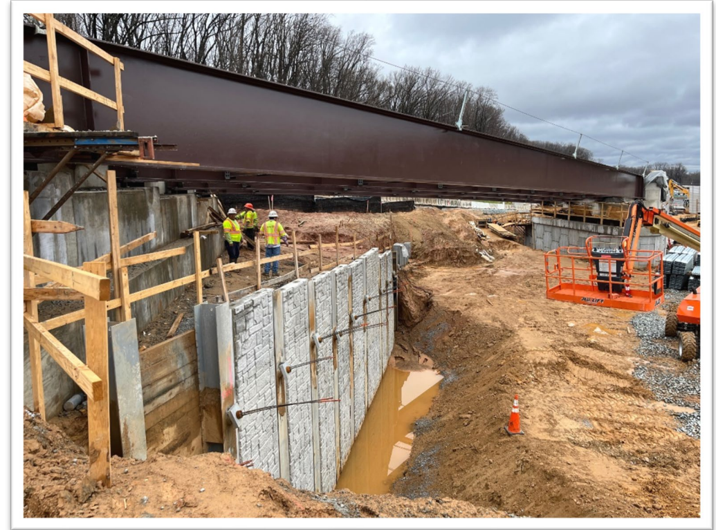
Four 100-ton girders were lifted into place for an overpass for the future southbound I-495 to Georgetown Pike ramp (February 2024)
