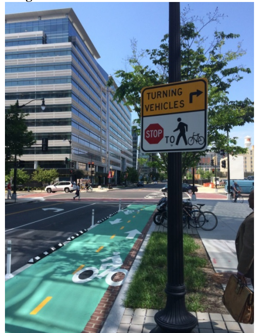
Figure 6: 1st Street NE Protected Lane
