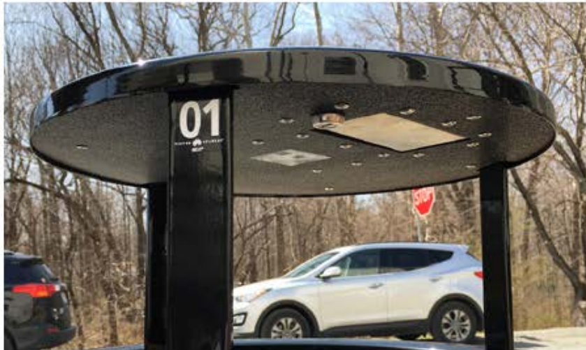
Relay sensor with replaceable batteries embedded within dome lid
