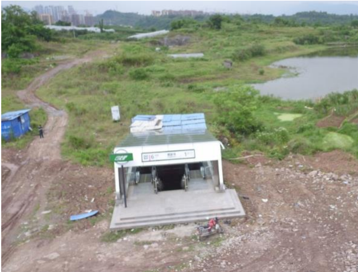
Caojiawan Station, Chongqing
