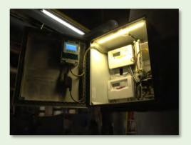
To monitor solar thermal system performance, Skyline employs the "SkyBox", a component delivered by a domestic hardware manufacturer and integration company according to Skyline's design and specifications. SkyBox is a turnkey component with enclosure and commodity hardware including the system sensor monitor, data backhaul computer, networking equipment, and power- and revenue-grade energy calculators.
