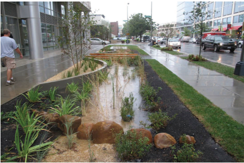
Rain garden: District of Columbia
