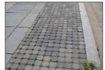
Permeable pavement: District of Columbia
