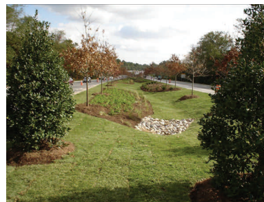
Bioretention in median: Prince George's Co.
