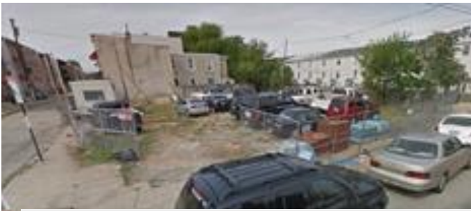
The North 16 th Street site in Philadelphia, PA under construction for Habitat for Humanity
