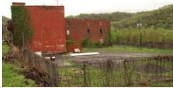
Hinton Ice House in Hinton, WV which will be part of the Rail Yard District
