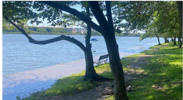
Figure 33. Flooding during high tide at the Tidal Basin in Washington, DC.
