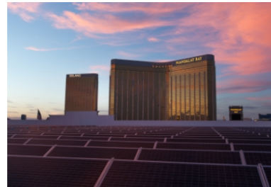
Photo Credit: NRG Energy
