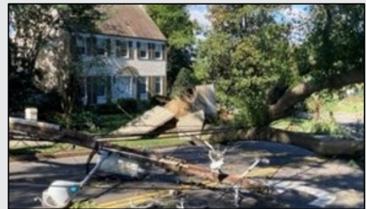
Figure 3: Fallen trees and broken power lines after the severe storm in 2023 ( Washington Post ).
