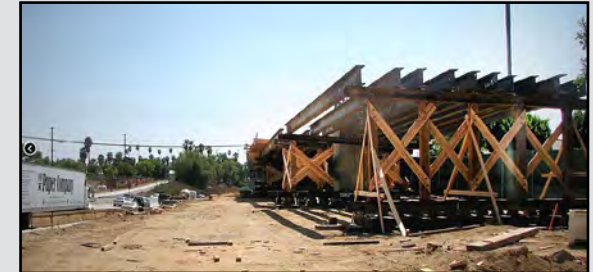
California is using GO bonds for transportation improvements.
