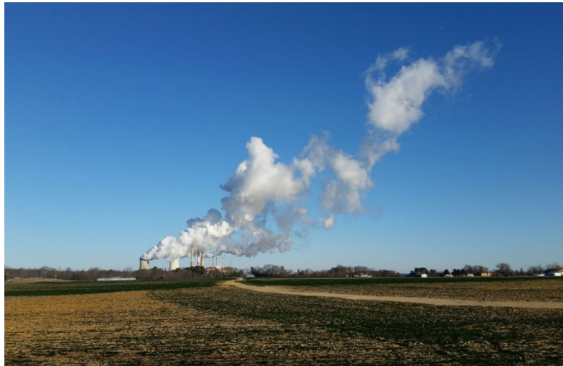
Chalk Point Power Plant in southern Maryland (Allie, Flickr)
