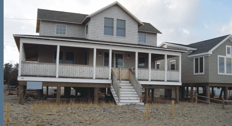
Example of Pile Foundation, Saco, ME. Image by P.A. Slovinsky, 12/2009.
