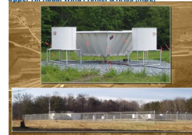
Upper-Air Radar Wind Profiler & RASS (MDE)
