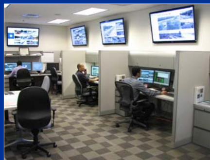
Signal Operations Center (SOC)
