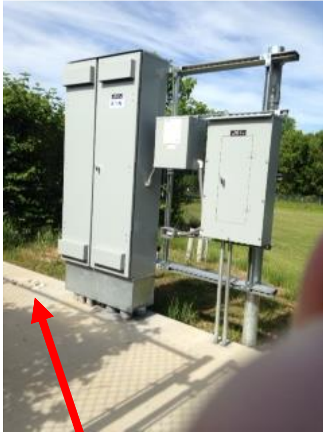
Conduit for future 10 stations capped off
