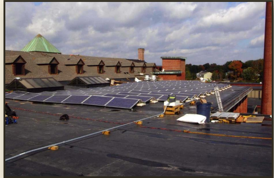
Low-profile solar panels installed on a large flat roof
