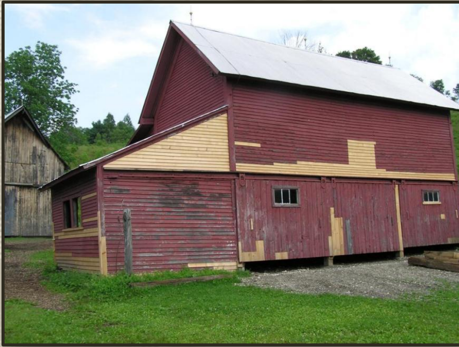
Howe Farm Creamery Building, VT
