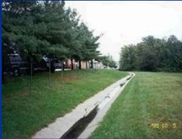
Untreated oily runoff from a parking lot
