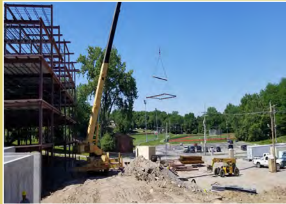
Top: After conversion Above: During conversion Credit: Fouch Brothers LLC
