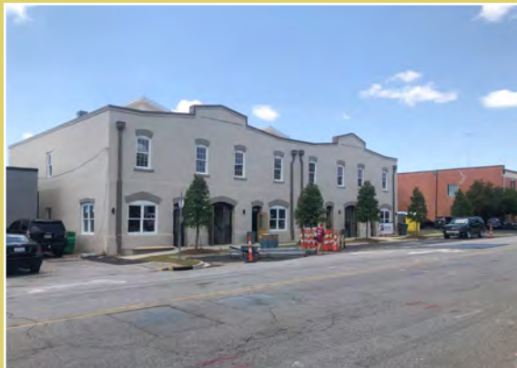
Top: Kitchen after conversion Above: Exterior after conversion Credit: Gavin Design Group
