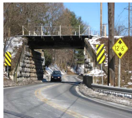
Restricted clearance CSXT and MD 75
