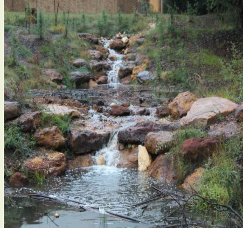
Cabin Branch RSC project
