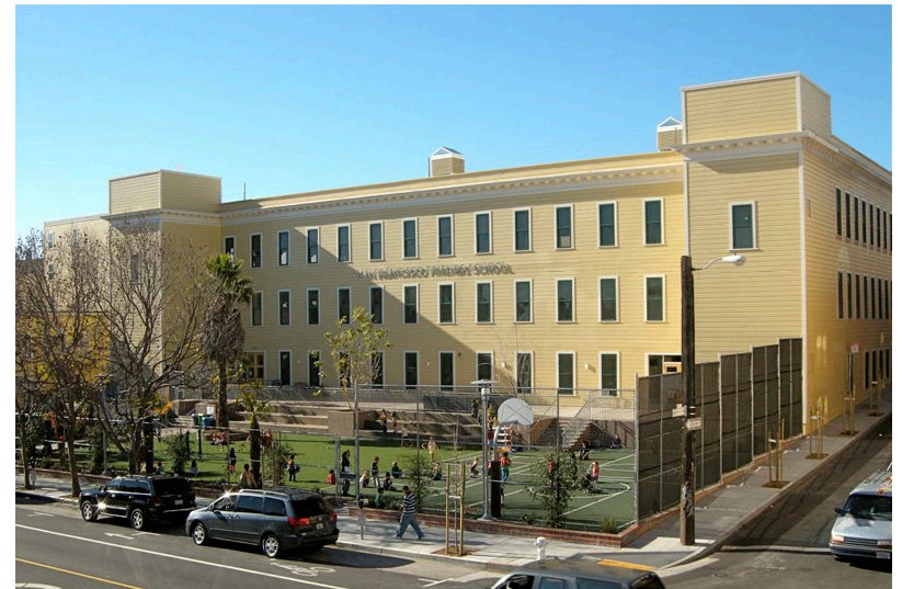
San Francisco Friends School – Solar@School Lead
