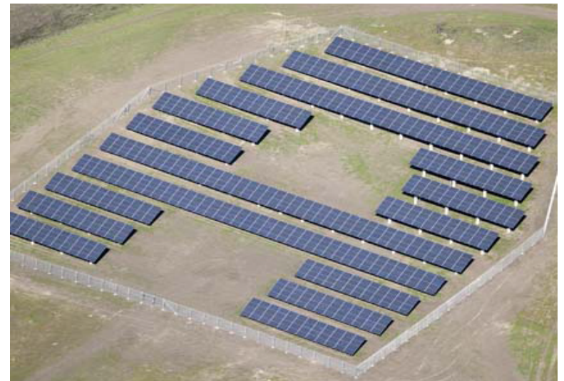
Solar School Pride - Athenian School 221 kW PV install, Danville, CA
