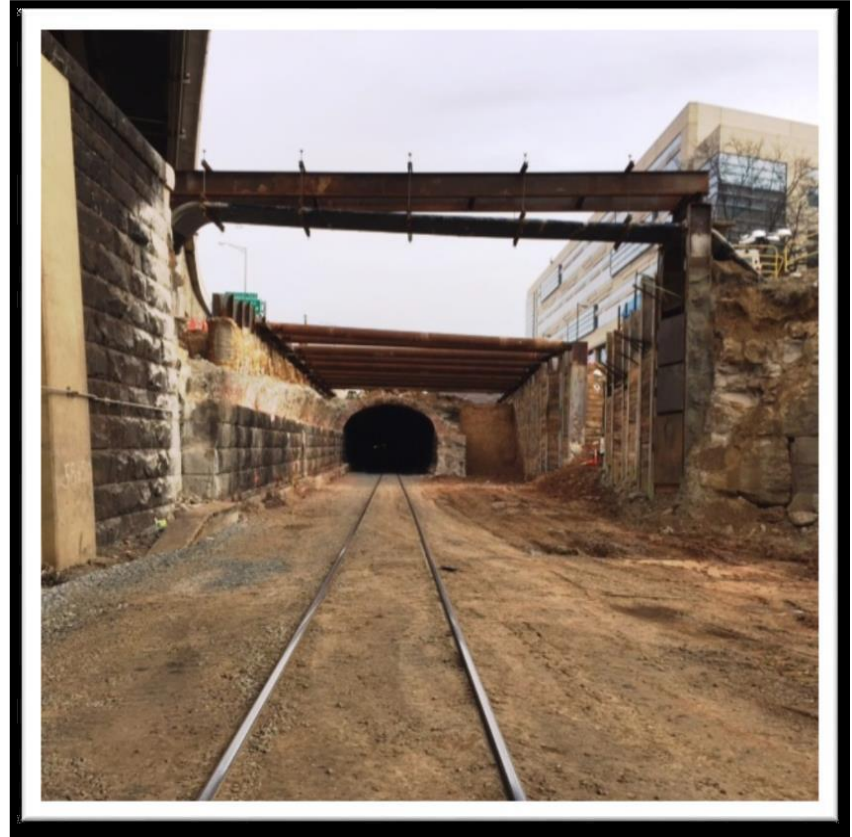
February 12 th Progress Photo (looking east)
