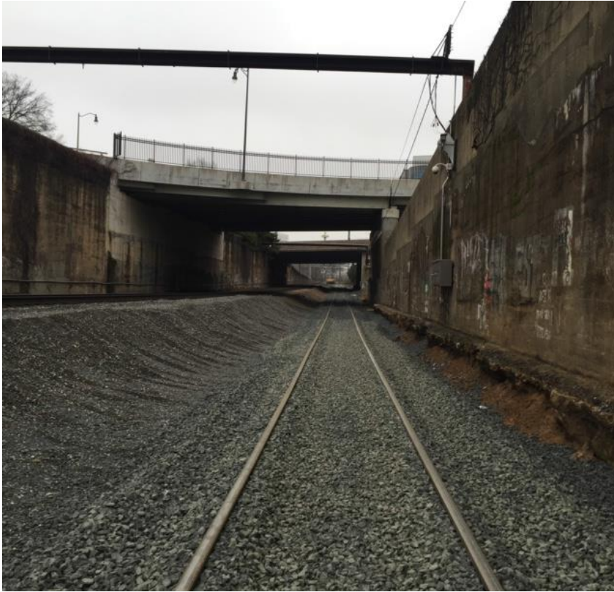
Track 1 Lowering Track Construction Complete
