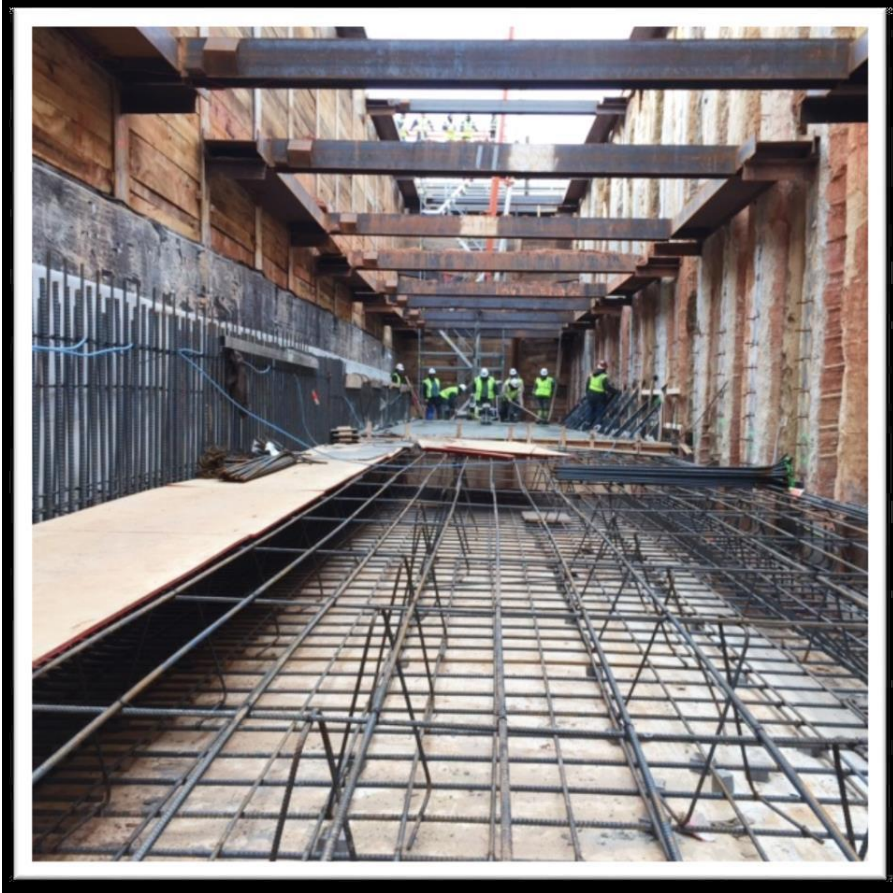
First Tunnel Invert (floor) concrete pour in the 400 Block—February 12 th (looking west)
