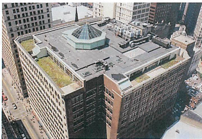
Left: Roof of the rehabilitated department store building with of green roof sections. Right: The tall parapet conceals the plantings and the penthouse from the street below.
