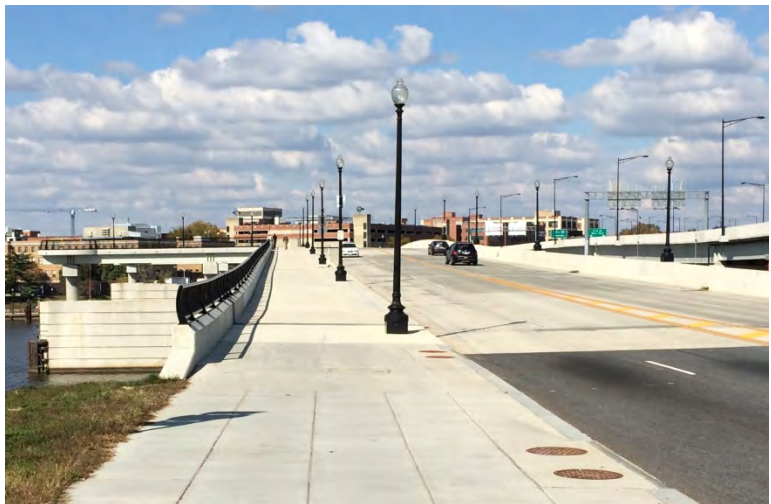
Figure 10: 11 th Street Bridge
