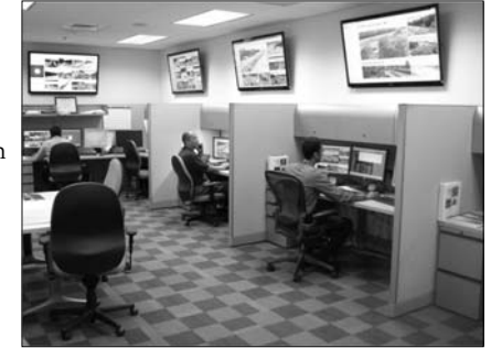
Signal Operations Center (SOC)
