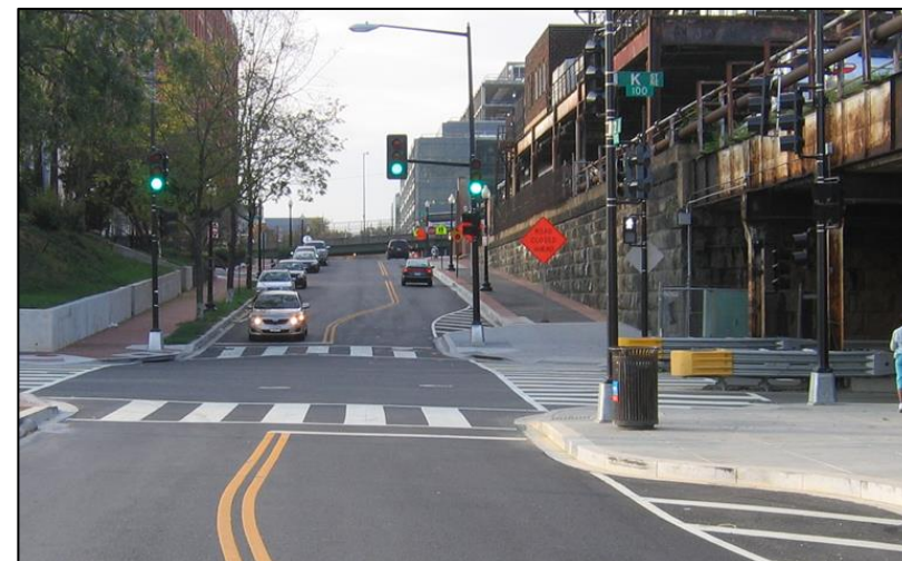
Concrete Curb Extension
