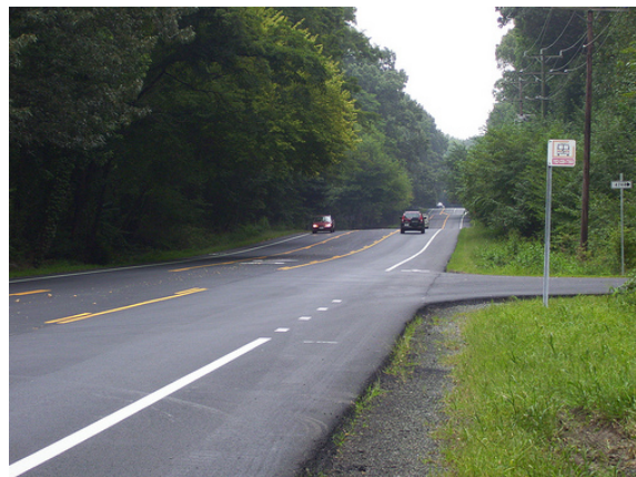
Figure 48: Lawyers Road After Road Diet/VDOT
