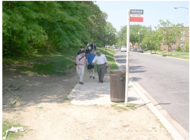
Figure 4: Missing Sidewalk/TPB/Michael Farrell
