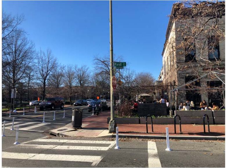
Figure 32: Flexpost Bulbouts/TPB/Michael Farrell
