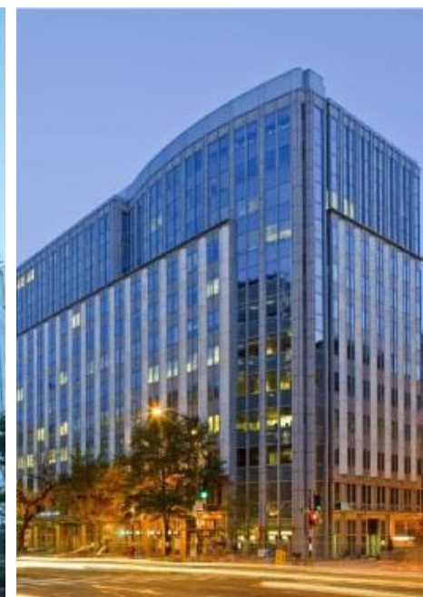
Millennium Building Tower Companies 20% energy savings $201k cost savings
