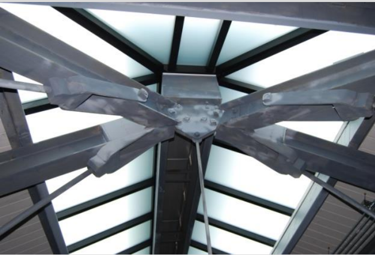
View of Skylight from below
