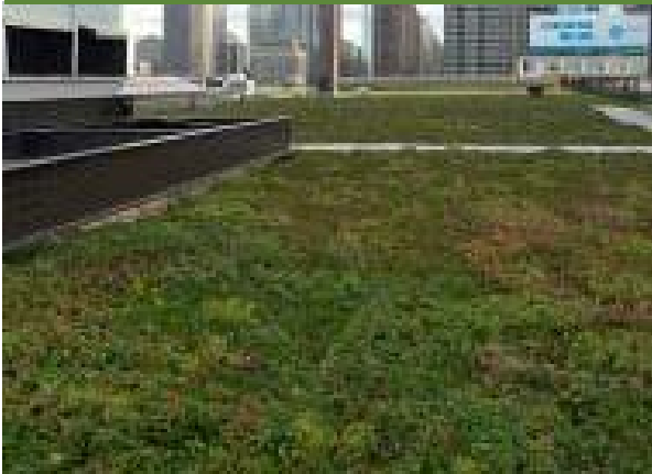
PECO Building, Philadelphia, PA
