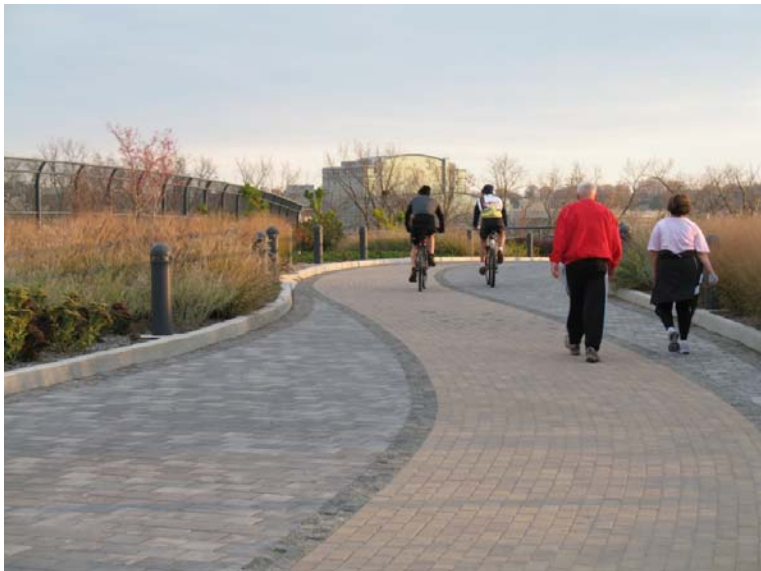
Figure 9: Woodrow Wilson Bridge Trail
