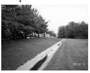
Untreated oily runoff from a parking lot
