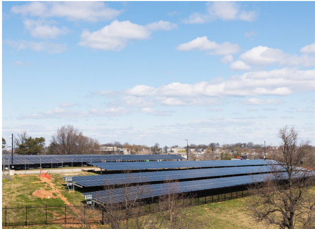
Brentwood Water Reservoir
