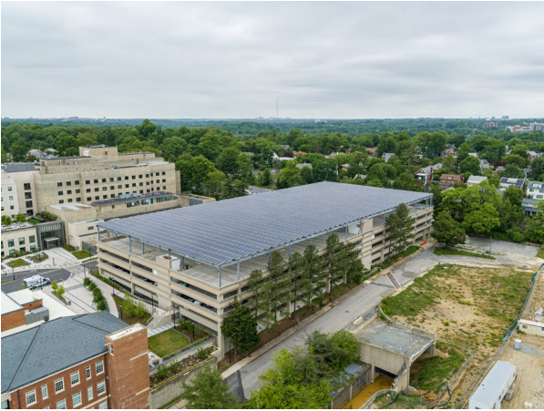
Children’s National Research & Innovation Campus at Walter Reed
