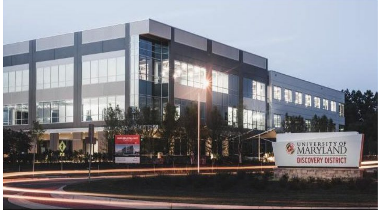
5801 University Research Center Court Riverdale Park North - UMD 75,000 sf office LEED Gold
