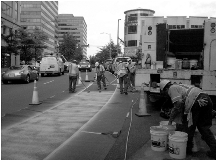
Workers paint green bike lane in Clarendon. Photo by BeyondDC/Flickr.
