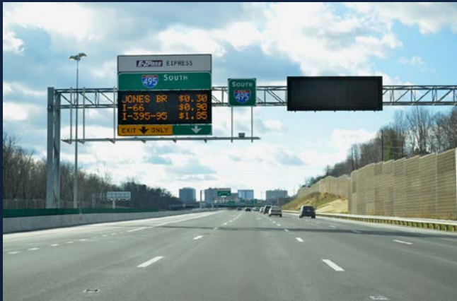
I-495 HOT Lanes (Opened November 2012)
