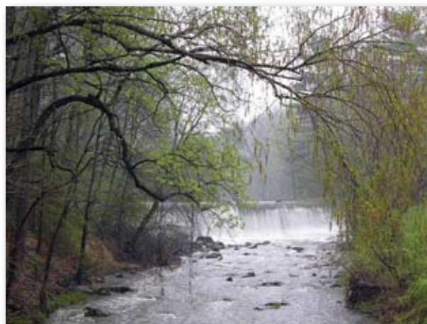
Burnt Mills Dam, Maryland.
