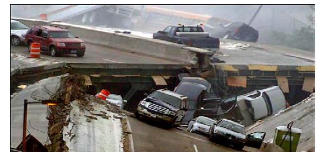
The 35W Bridge 2007
