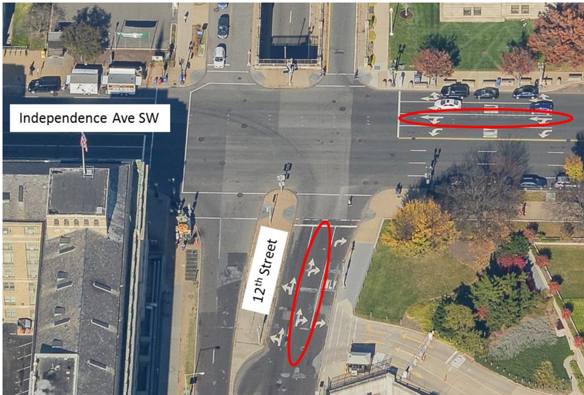
Photo: aerial view illustrating lane configuration changes recommended at 12 th and Independence.
