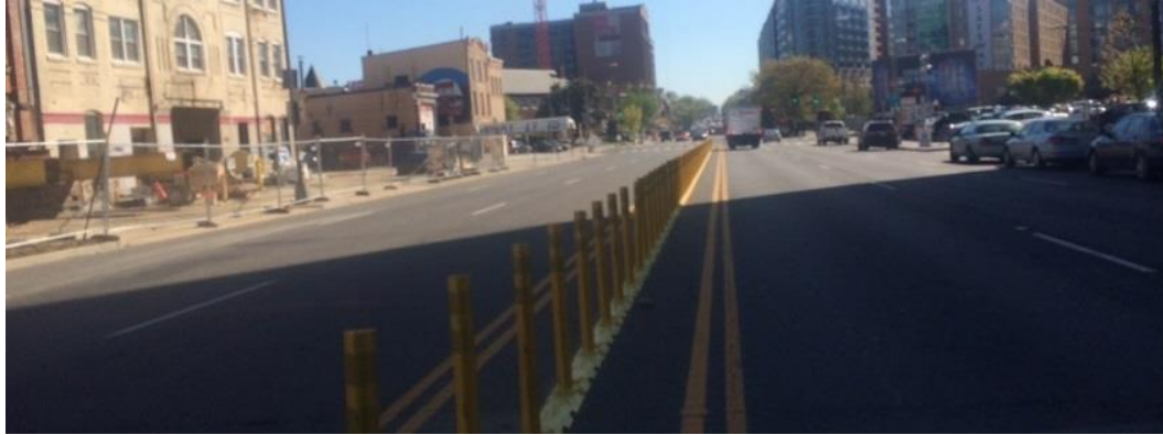
Photo: Flexible tubular post on New York Avenue. These are recommended on K Street NW to prohibit midblock left turns into the service road access points
