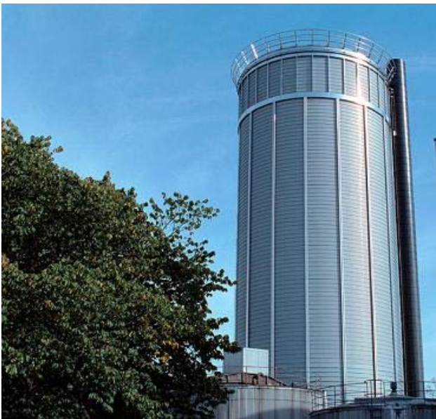
Figure 15. Hot Water Accumulator
