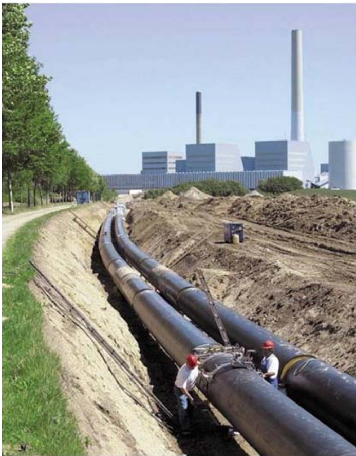
Figure 6. Long Distance Heat Transmission
