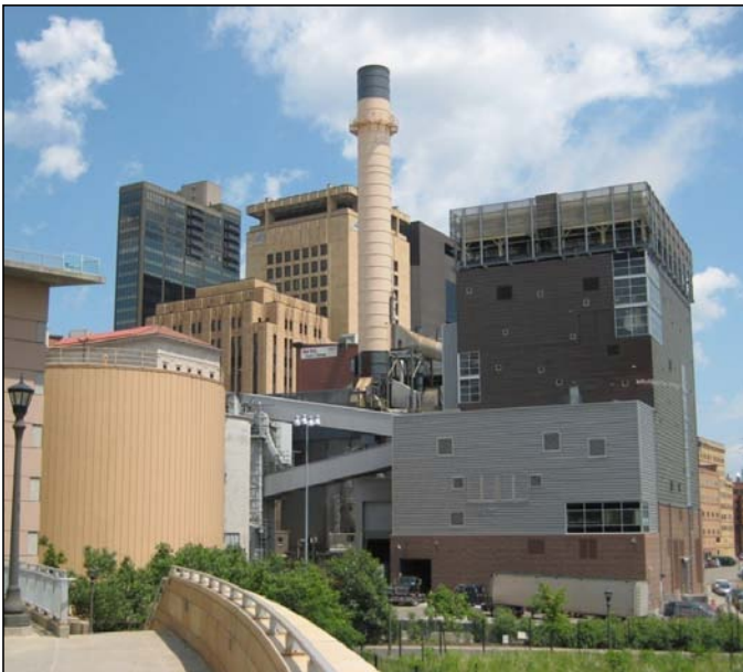
Figure 8. Biomass CHP Plant in Downtown St. Paul, Minnesota, USA
