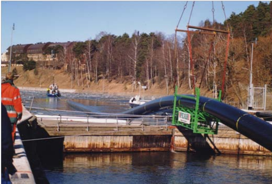
Figure 13. Installation of Polyethylene Pipe for Deep Water Cooling from Lake Mälaren, Sweden
