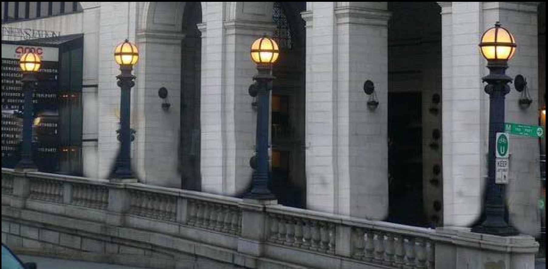
Retaining Wall and Lamps at First St.
