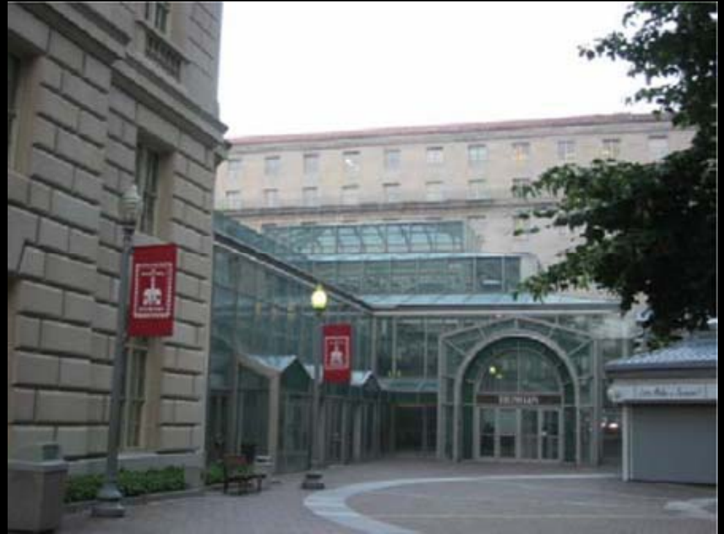
Tent Structure, National Mall, Washington DC
