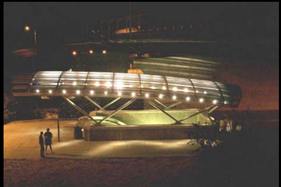
Metro Entry, Washington DC
