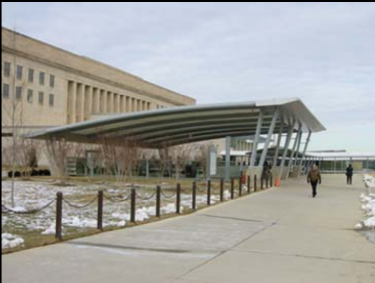
Pentagon Transit Facility, Washington DC
