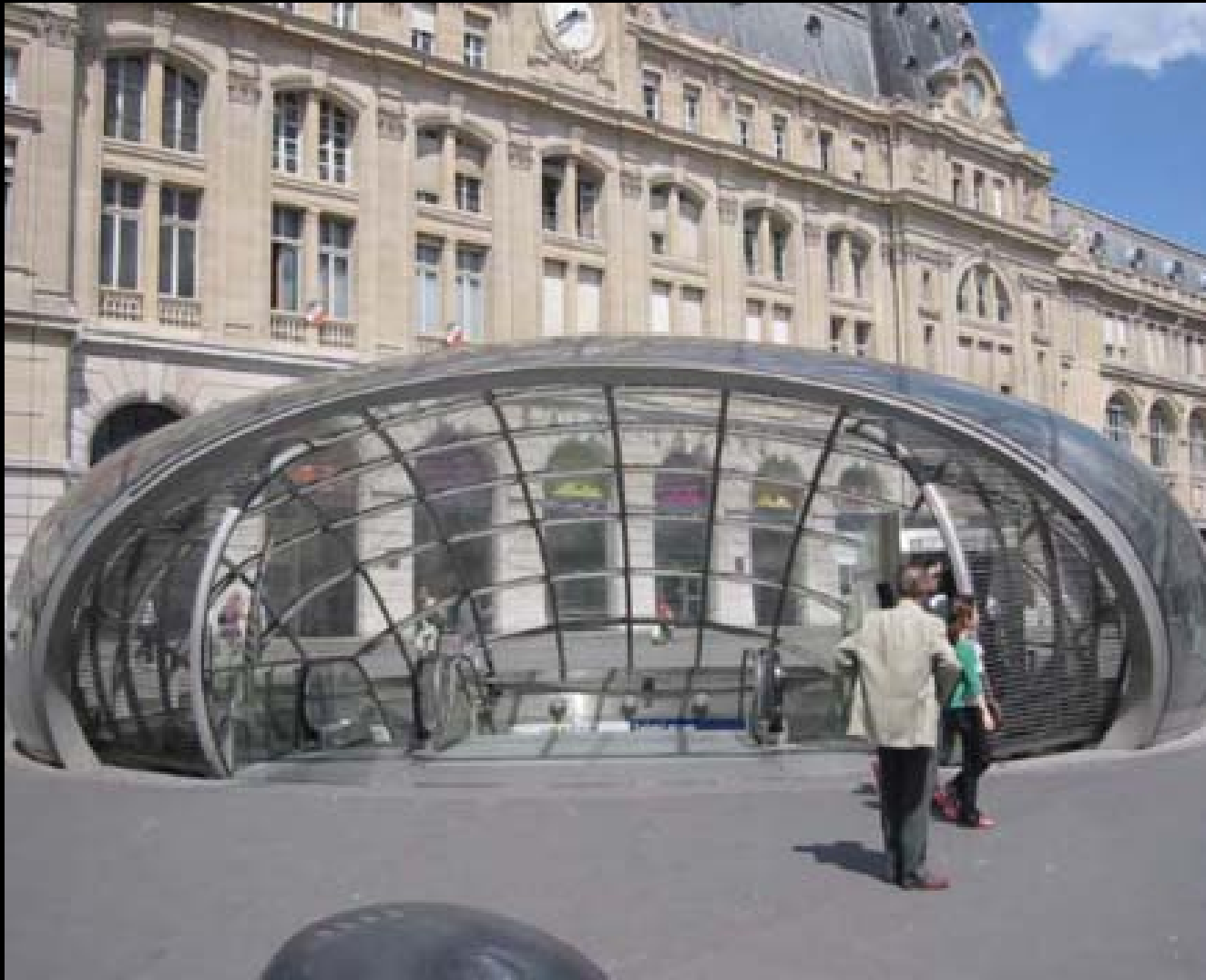
Underground Entry, London
