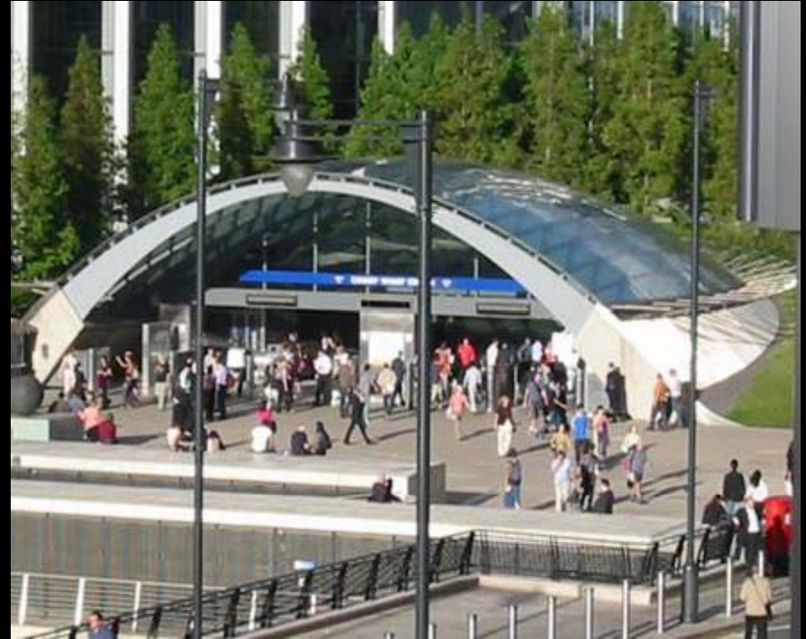
Underground Entry, Canary Wharf, London
