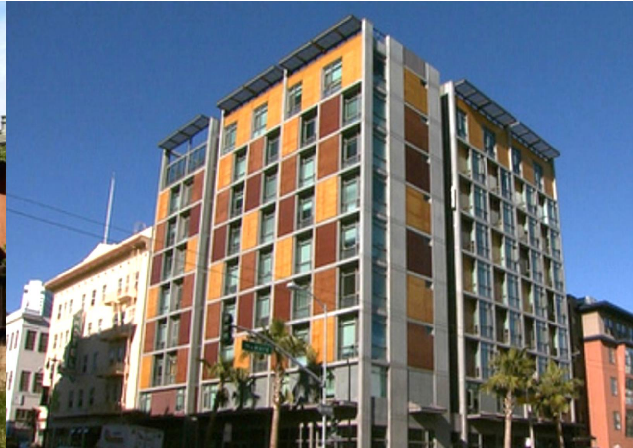
Plaza Apartments, San Francisco Supportive Housing
