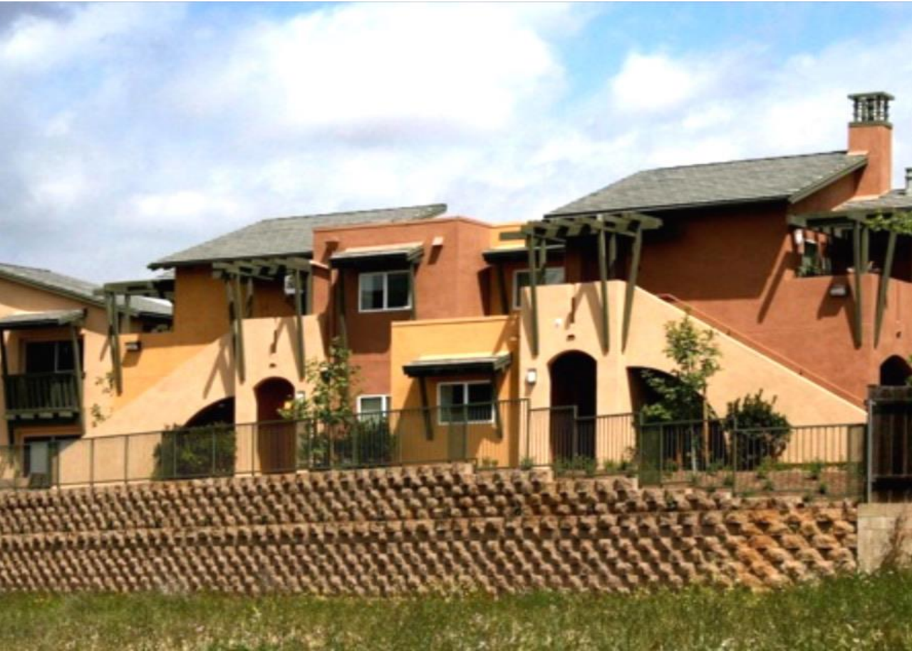
Solara, San Diego Zero Energy Affordable Housing
