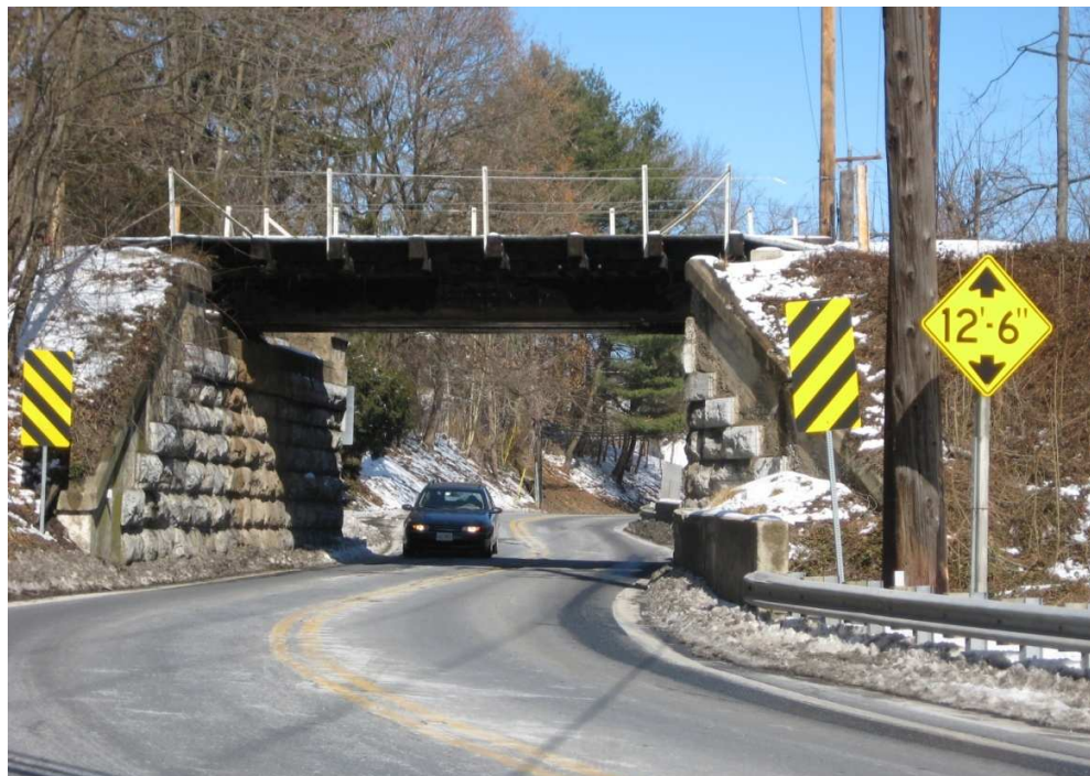
Restricted Clearance for Trucks Under CSXT Bridge on MD 75
