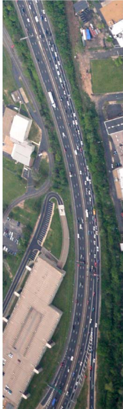
Figure A5: Aerial Photo of the Entrance Ramp to D.C. 295 from Firth Sterling Ave
