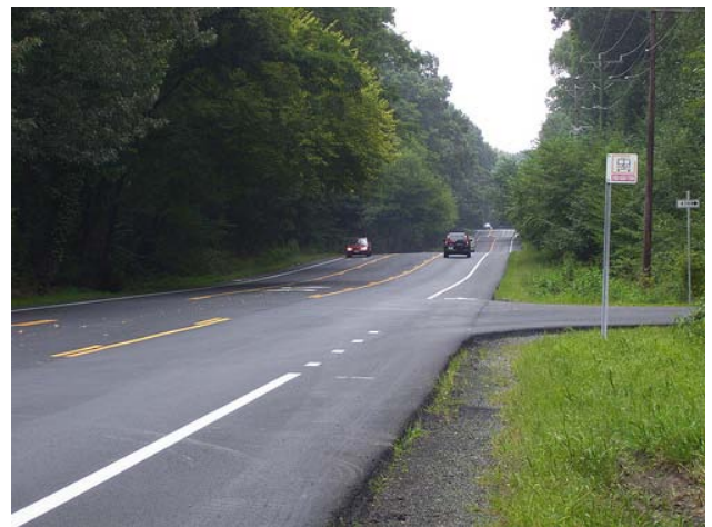
Figure 14: Lawyers Road After Road Diet
